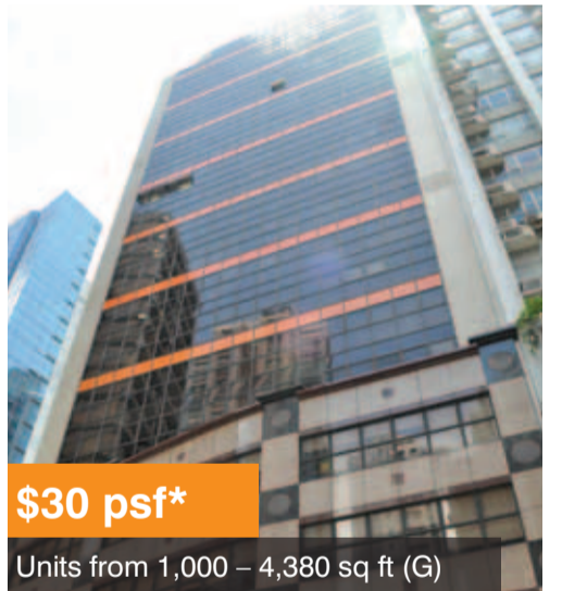
$30 psf* Units from 1,000 – 4,380 sq ft (G) 299 Queen's Road Central Sheung Wan
